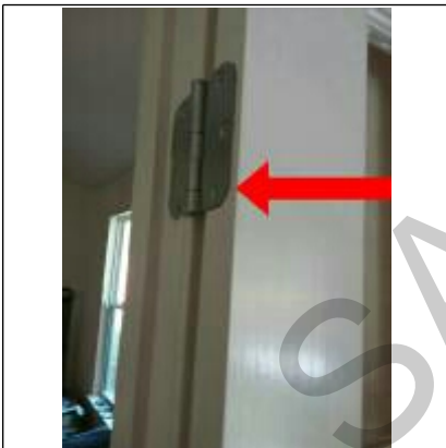
Hinge bind prevents closing tightly
